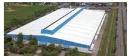
Fujitsu General (Thailand) Co., Ltd. (Thailand) FACTORY-2
