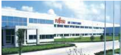
Fujitsu General (Shanghai) Co., Ltd. (China)
